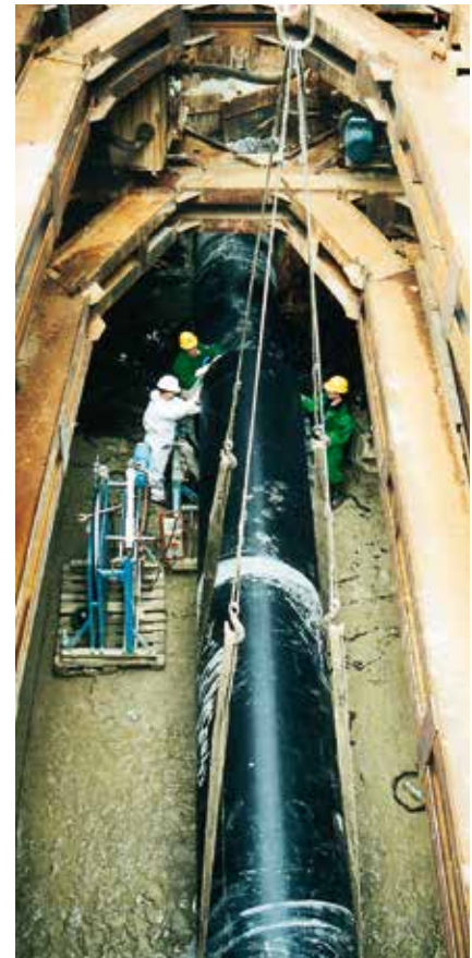
Long pipe relining
